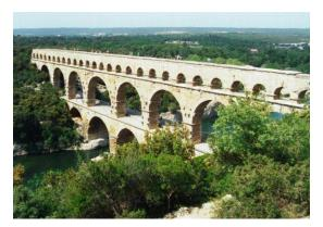
plumb bob and protractor was placed in the channel to measure the correct slope. When an aqueduct crossed a depression over 150 feet deep, a gravity pressurized inverted siphon was used to force the water uphill, as used by hydraulic engineers today. Arriving in a city, the water flowed into large holding tanks to let mud and
