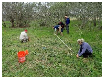
Putting the 3-4-5 rule into action to lay out perpendicular and parallel points to original line (photo by John Rich)
